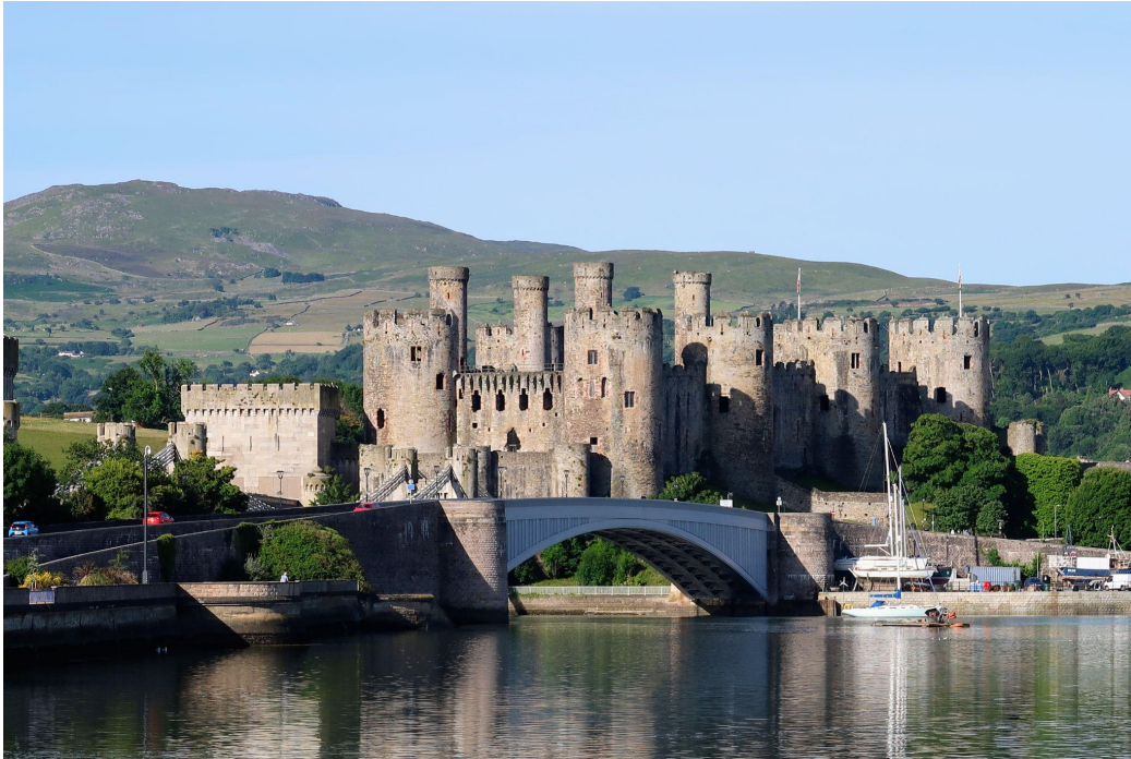
A view from the water of Conwy Castle, a short drive from Bodysgallen Hall & Spa. Photo credit - Wikimedia Commons
